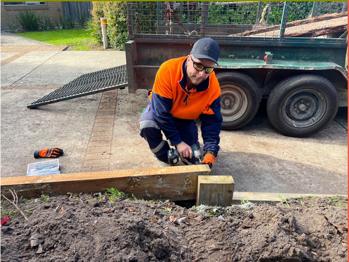
Nick Ray (EWD) building a retaining wall at DFFH site
