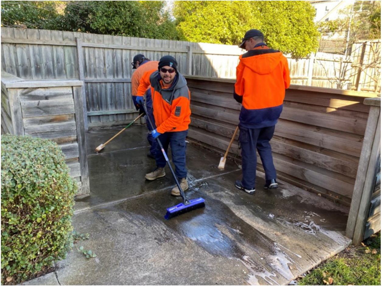
DFFH Site in Cheltenham Paul Ricupito (EWD), Matthew Bennet (EWD) and Robert Tost (General Labourer) cleaning site
